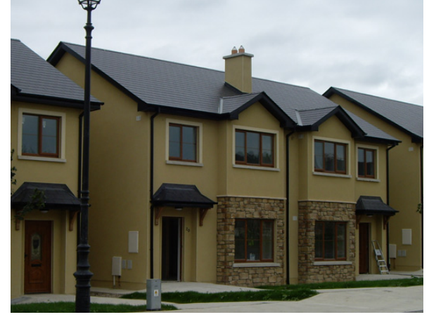
Cygnum Timber Frame Houses (prefabricated off site)
