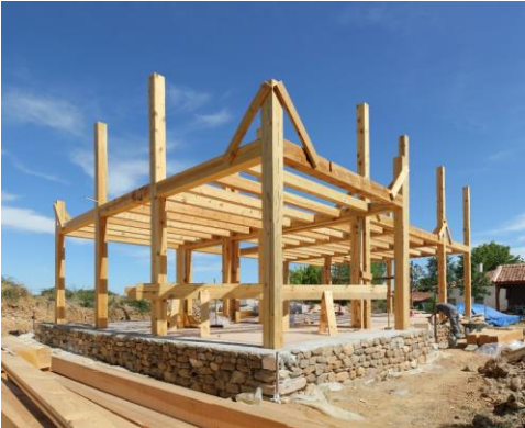
Post-and-beam house under construction in Barahona (Guadalajara) Novadomus Hábitat
