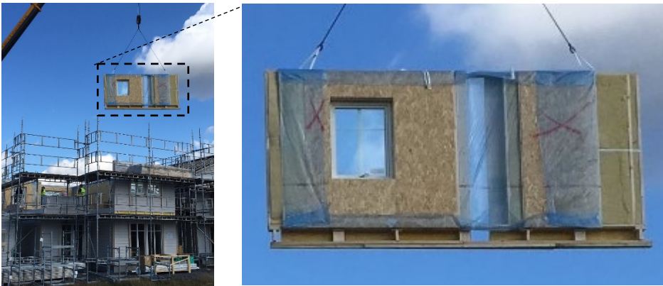
Figure 11 Exterior wall panel lifted in place during assembly, ends are left open to allow for screwing. Image: Derome
