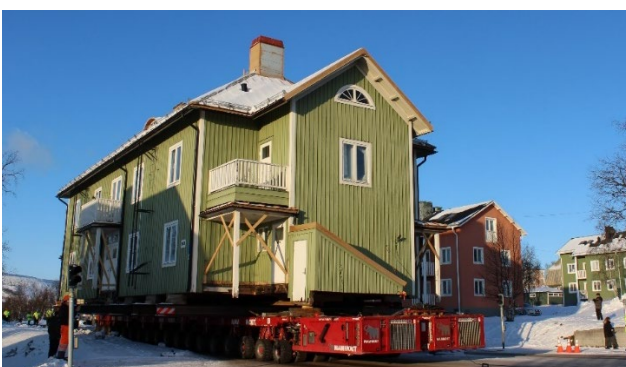
Figure 32 Buildings can be moved in their entirety as an alternative to demolition. The photo shows a two-storey timber building being moved in Kiruna. Image: Kiruna municipality
