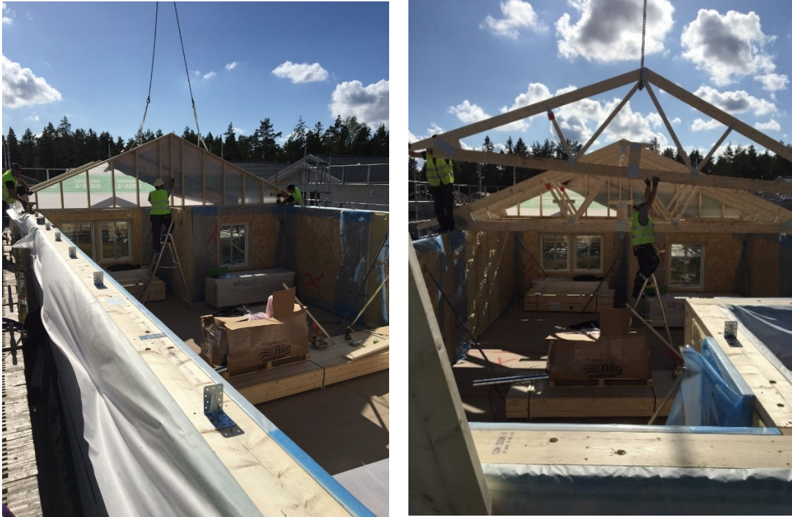
Figure 9 Angle brackets connect roof trusses to walls. The photos show roof trusses being installed. In this specific case, the assembly team has mounted the angle brackets before mounting the roof truss. Images: Derome
