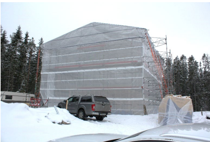
Figure 14 Weather protection. Methods and instructions for weatherproof deconstruction needs to be developed. Image: Andreas Videll, Derome
